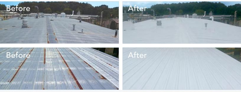
The metal roof pictured above was littered with rust and leaks, rendering the metal almost useless. On top of the rust and leaks, many fasteners had backed out and exposed holes in the roof. After priming the roof with P-130 Rust Inhibitive Primer, Pro-Eco Sil HS 3201 silicone coating was used to seal the roof, prevent leaks, hold fasteners in place, and improve overall performance. On top of all these benefits, the roof now has a 20 year warranty.
